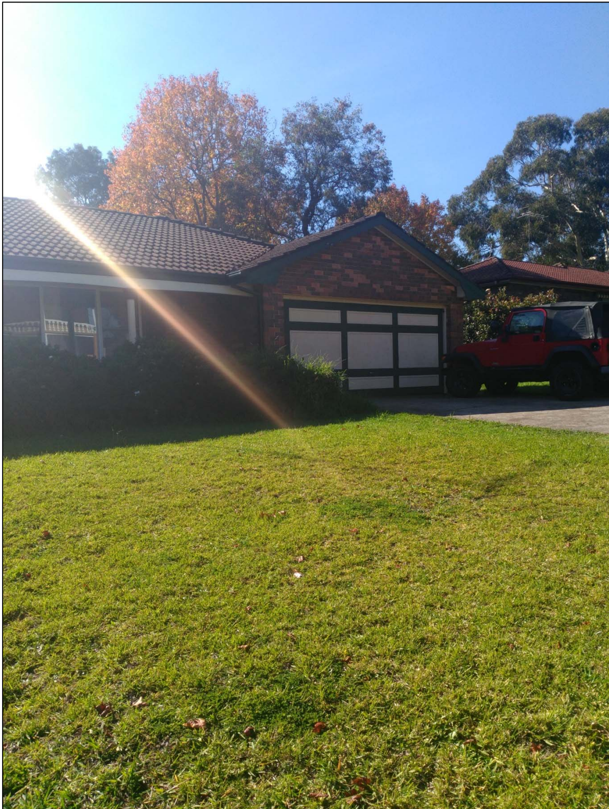
Photograph 4: Roof tiles were consistently used on buildings throughout the entire site. It cannot be discounted that they may contain fibrous asbestos cement material.
